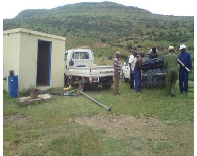
Borehole pump installations.
